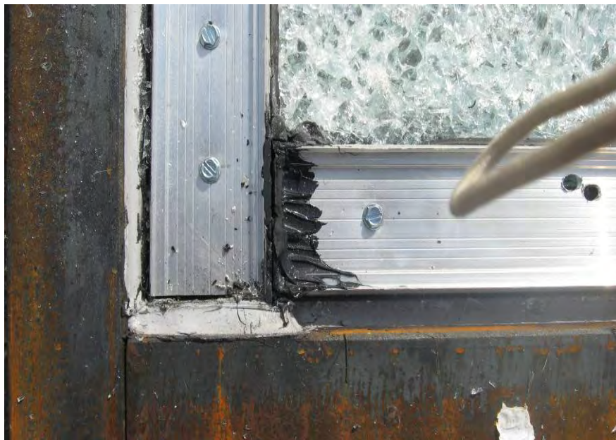
Photo No. 10 Horizontal and vertical corner connection
