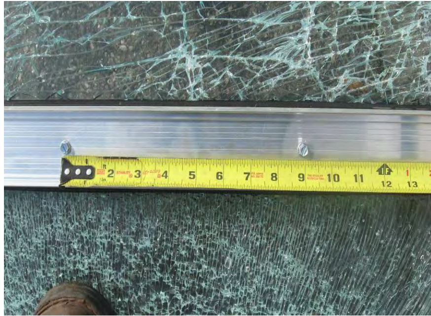
Photo No. 13 Fastener spacing on all pressure plates
