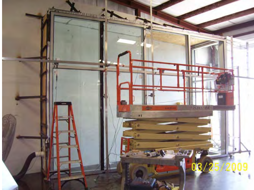
Photo No. 1 Overall view of aluminum curtain wall
