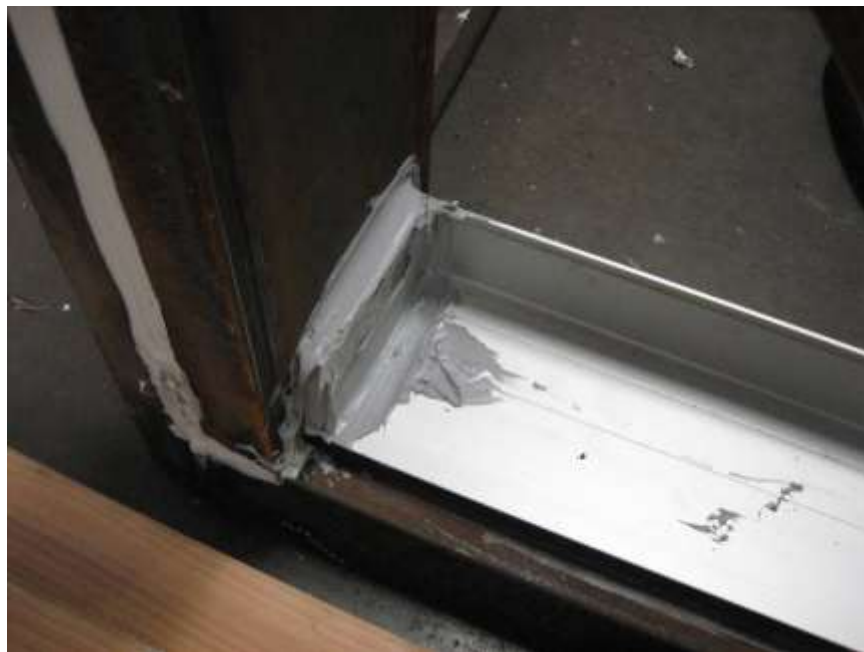
Photo No. 8 Specimens #1, #2, #3 Typical Corner Detail at Sub-Sill
