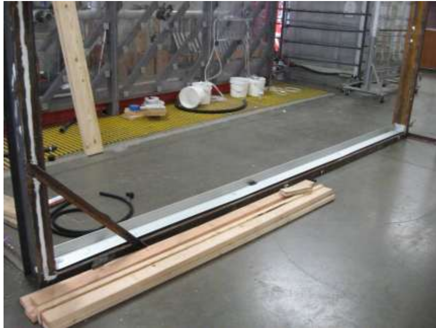
Photo No. 7 Specimens #1, #2, #3 Installation of Sub-Sill
