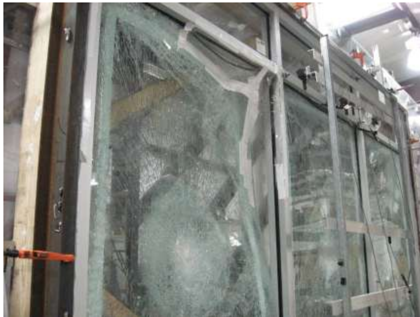
Photo No. 6 Specimen #1 Failure of glazing at upper right corner of specimen during TAS 203 positive loading
