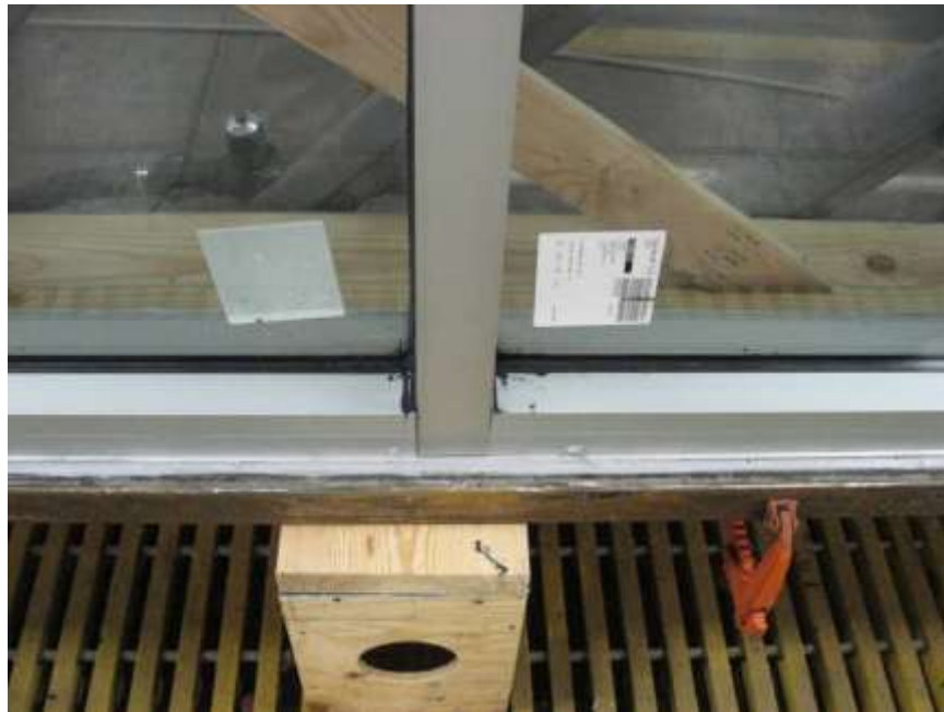
Photo No. 3 Specimens #1 and #2 Typical mullion detail at exterior
