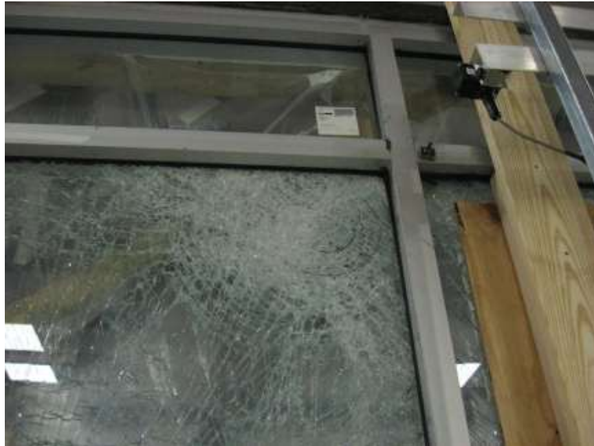
Photo No. 11 Specimen #R-1 Impact at upper right corner
