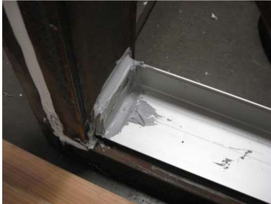
Photo No. 13 Specimens #1, #2, #3 Typical corner detail at sub-sill
