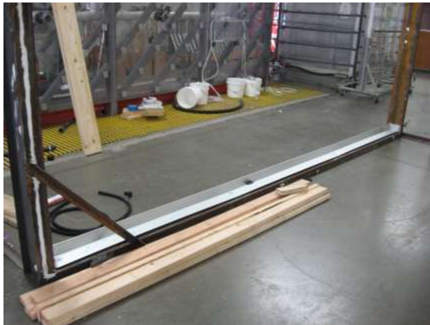
Photo No. 12 Specimens #1, #2, #3 Installation of Sub-sill
