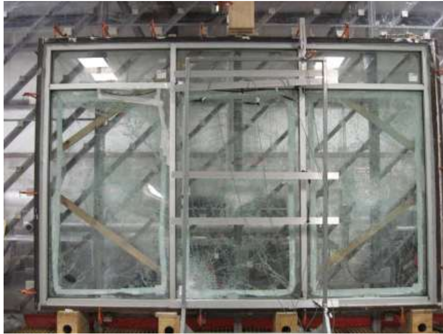
Photo No. 5 Specimens #1, #2, #3 Exterior view during TAS 203 cyclic loading; Specimen #1 at far left experienced a failure
